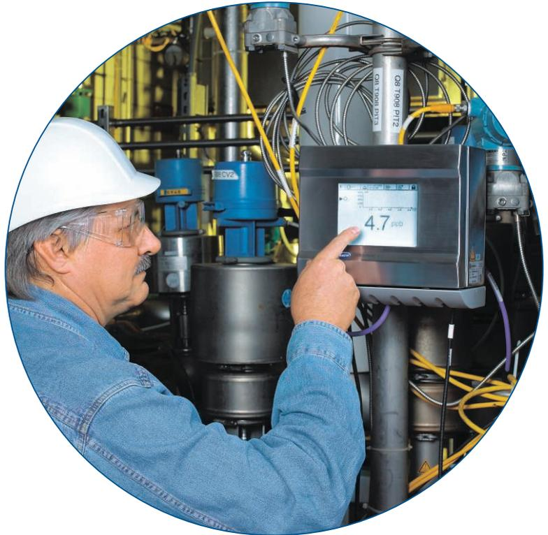
Controlling oxygen levels with the ORBISPHERE K1100 and 410 controller
